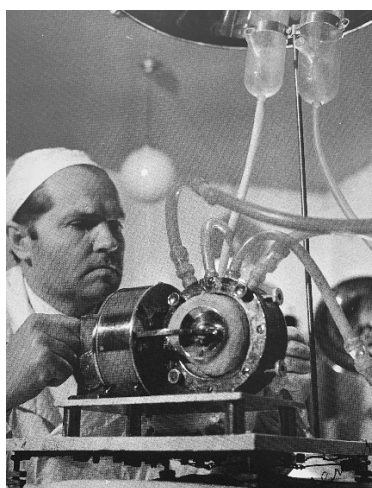
Fig. 4. Heart-lung machine designed by V.P. Demikhov and intended for a) revitalization of a cadaveric heart for the purpose of its transplantation; and b) resuscitation of those dying in ambulances. 1960s [1]
